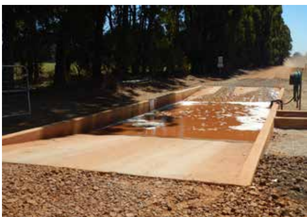
Figure 31: Vehicle dips are useful to disinfect low-risk vehicles that require access to your packing shed via your separation zone
