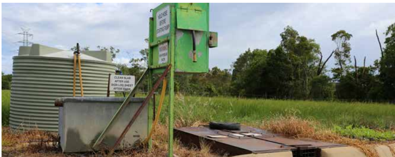
Figure 26: High-pressure hose and sump are essential elements of a wash-down facility
