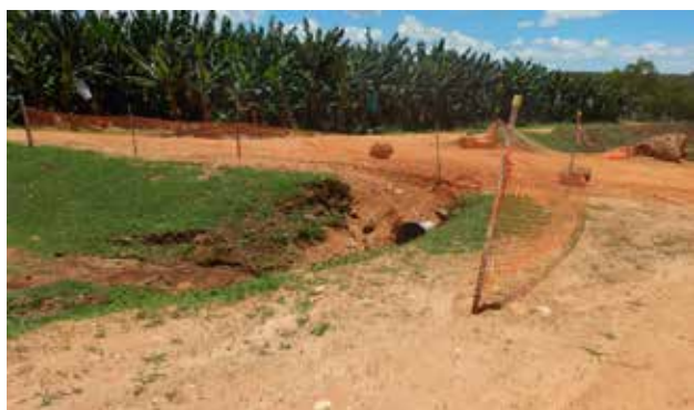
Figure 38: Example of earthworks and drains directing water away from a production area
