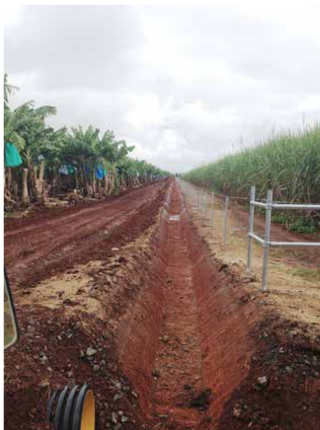
Figure 40: Drainage used to intercept water from neighbouring properties and divert water away from a production area
