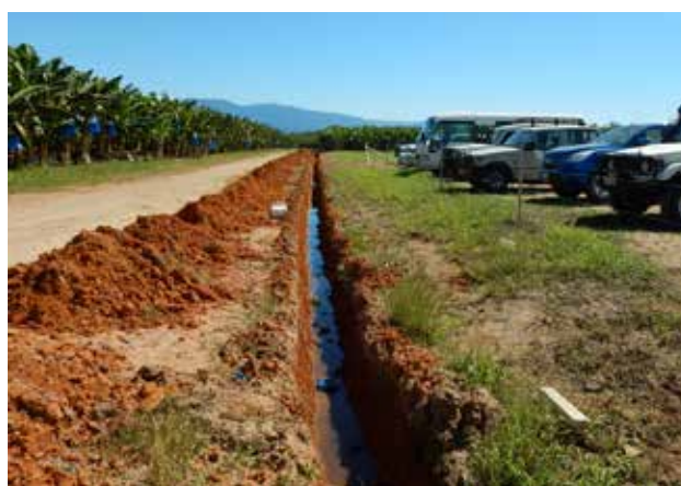
Figure 3: Drainage between zones to manage run-off water
